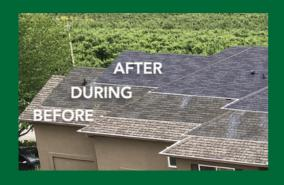
Once all prerequisites are addressed, we initiate the roof rejuvenation process. The product, precisely mixed at a 70/30 ratio with water, is applied by our skilled team using a low-pressure spray, ensuring an efficient and seamless application, covering up to 10,000 square feet per day. The product settles and cures within just a few hours, breathing new life into your shingles and restoring them to their original color and vitality, leaving your roof looking rejuvenated and like new.
